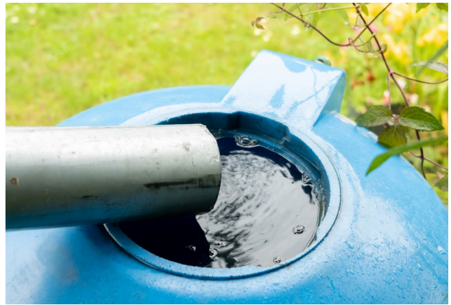
A tank placed under gutter downspout collects rain water.
