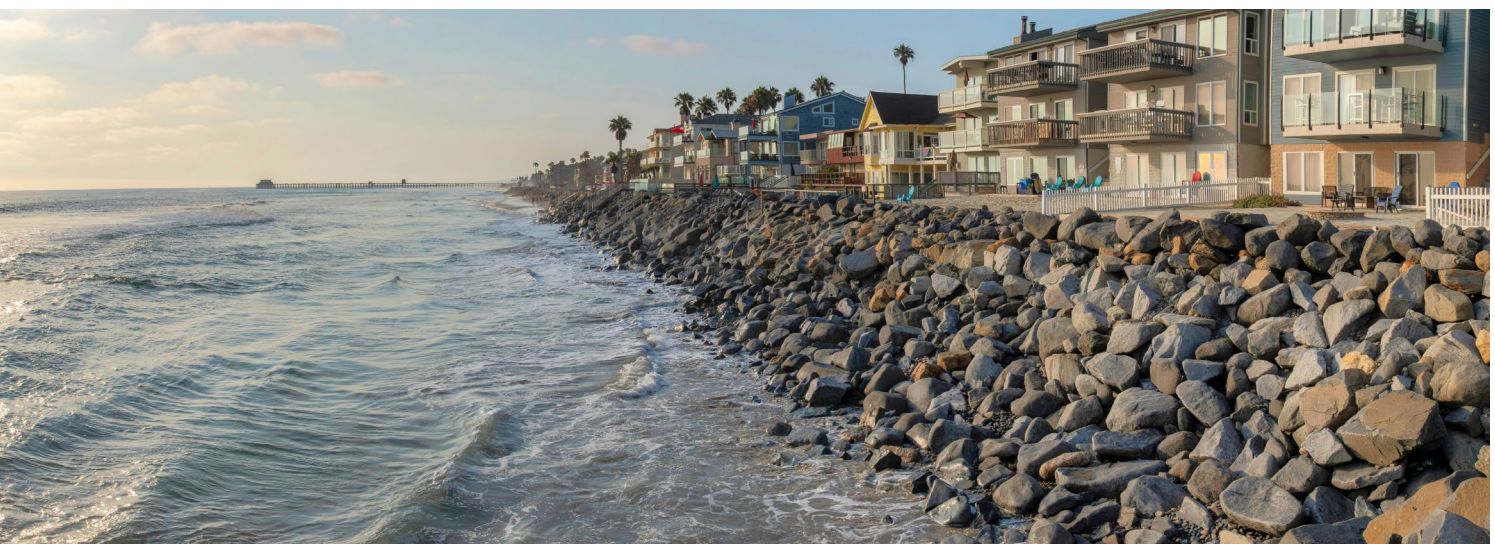
Armoring to protect ill-conceived coastal development is a primary contributing cause to coastal erosion and shrinking beaches, as it fixes once dynamic shorelines, and cuts off a replenishing sand supply.
