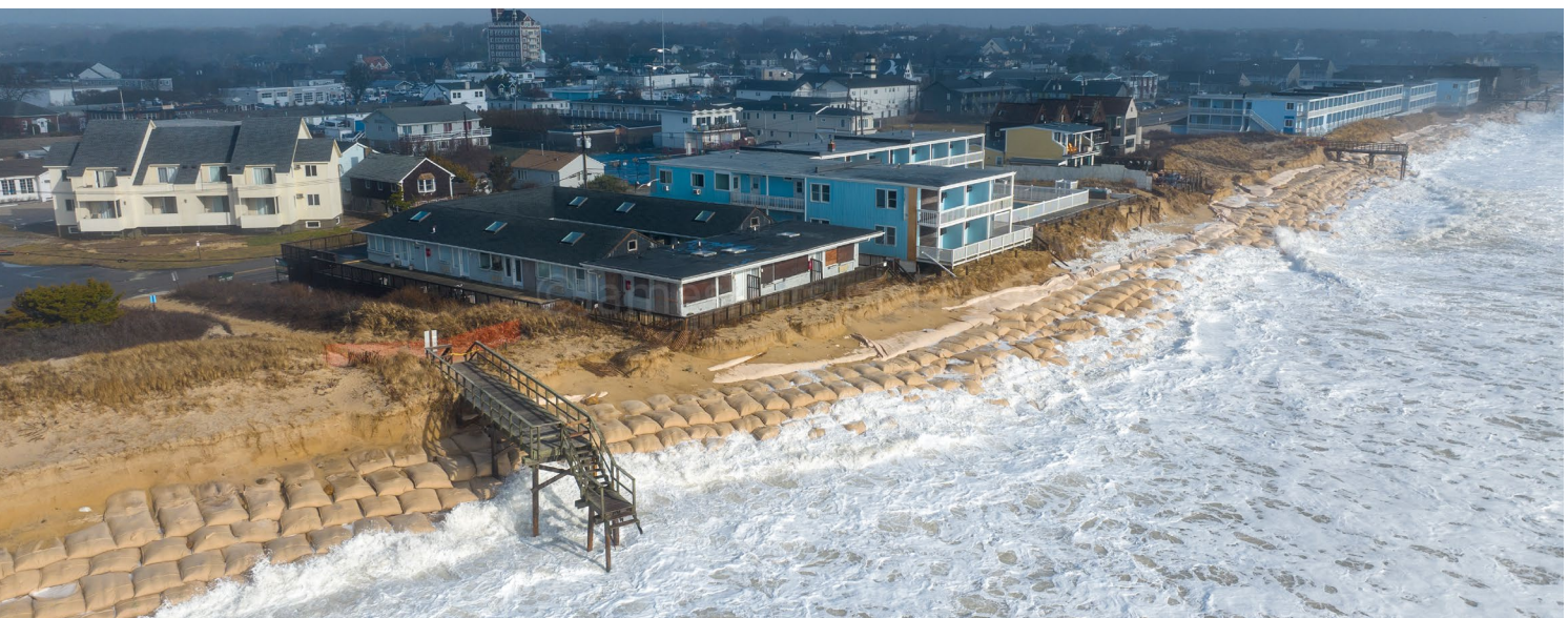
Extreme weather threatens properties along the coast of Montauk, NY, demonstrating the negative effects of using short-term armoring as a long-term solution. © James Katsipis
