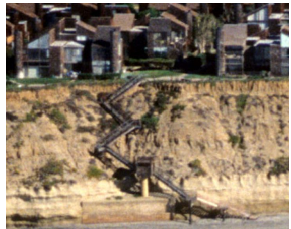
1989 8 - new staircase relies on seawall
