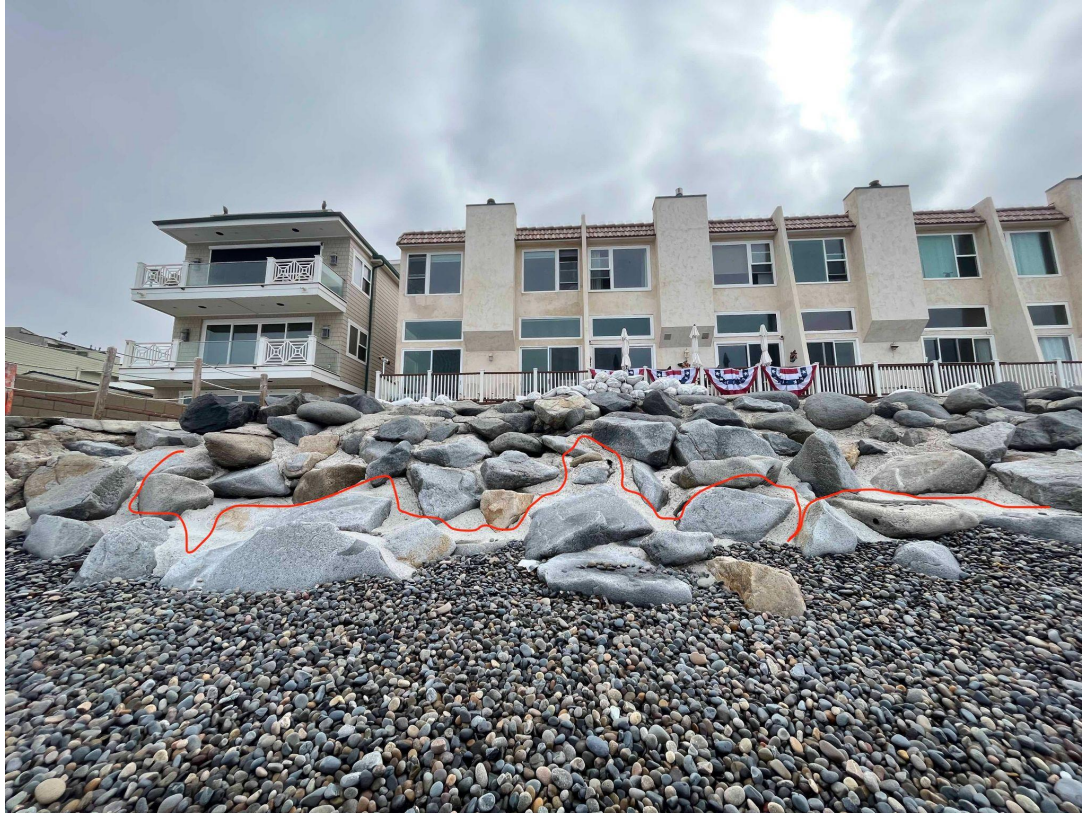
The red line traces concrete grouting
