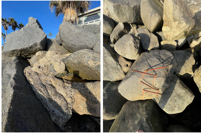
The presence of concrete grout and rebar
