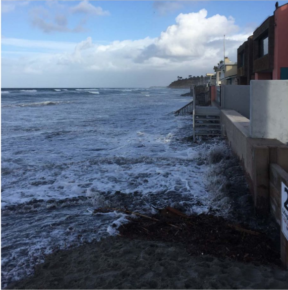
Overtopping in Del Mar, 3/8/16
