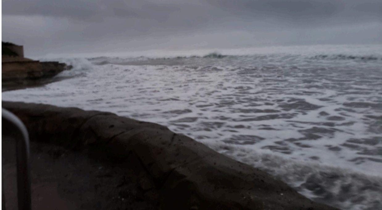
Flooding of beach access to South Cardiff State Beach and front of Steinberg Seawall as observed on January 18, 2019.
