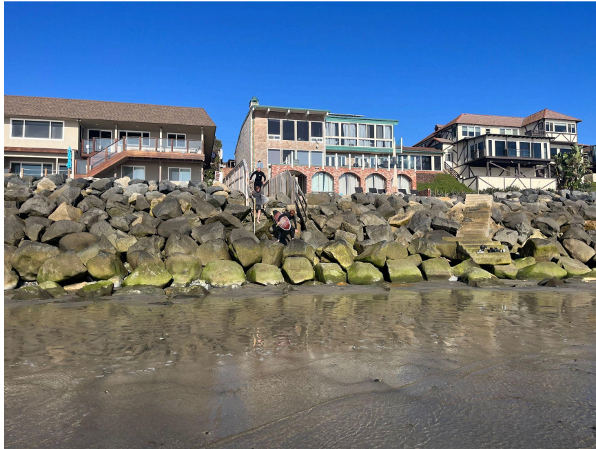
Young surfers negotiate privately-owned riprap that blocks public access in South Oceanside. Photo taken at negative low tide (usually there is no beach to access, note the absence of dry sand and moss on the riprap).
