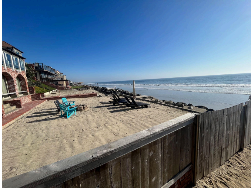
The adjacent properties to the South enjoy perched, private beaches made possible by their revetment atop public tidelands. Photo taken at negative low tide.
