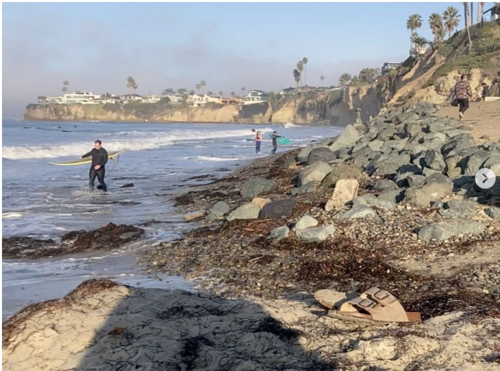
The ocean reaches the toe of the revetment during annual King Tides (2022)
