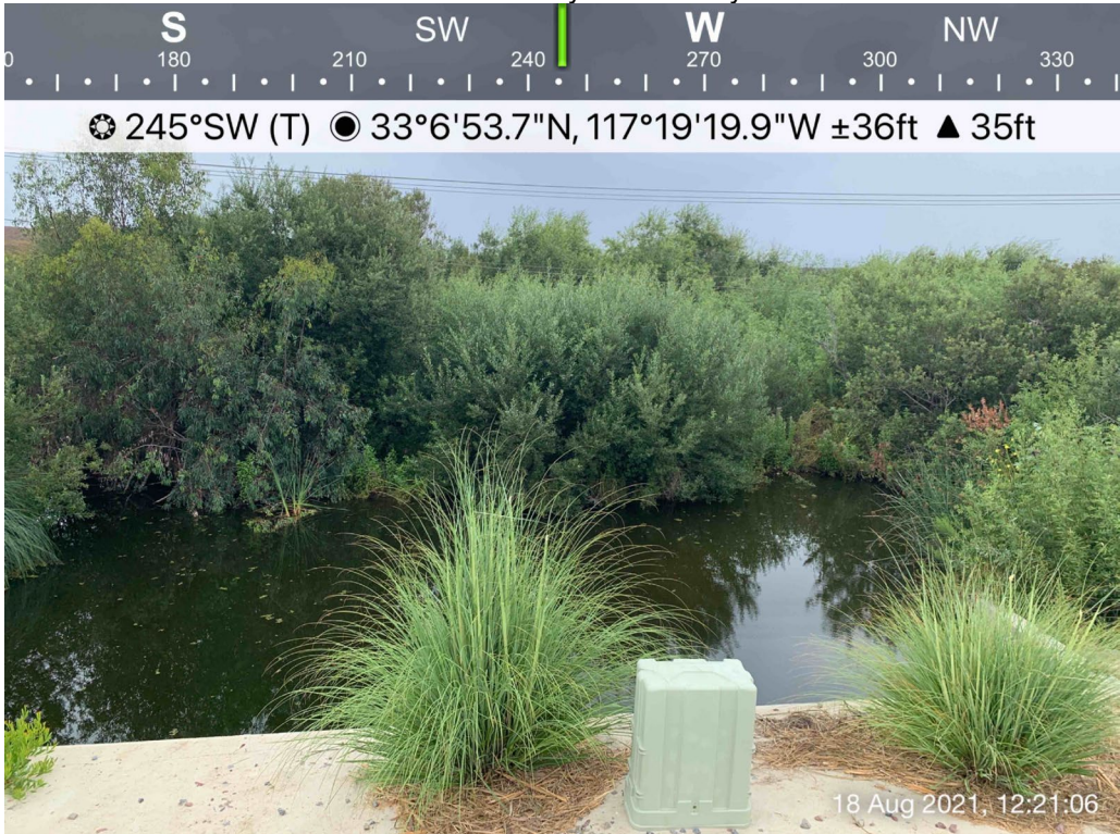
Photo 14. Dense arroyo willow surrounded the scour pool at the large Avenida Encinas culvert outlet.
