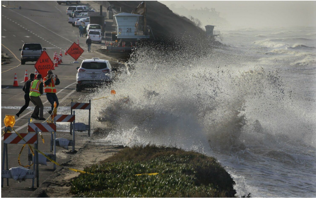
Photo 2. Coastal Flooding within the Project Area (source: City of Carlsbad)
