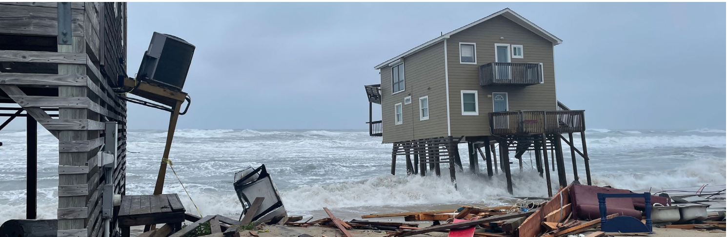
A home in North Carolina collapses into the sea due to coastal erosion and rising sea levels. © Cape Hatteras NPS / National Park Service
