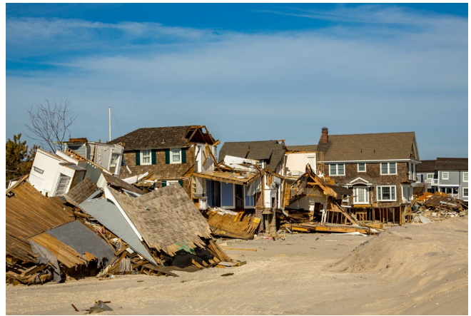
Hurricane damage to beach homes on the New Jersey shore.
