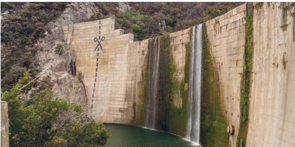
Abandoned and obsolete Matilija Dam and outbuildings in Ojai, California.
